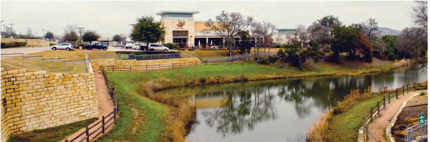
Water feature provides a dual purpose: stormwater management and a natural amenity along the Hill Country Galleria Trail
