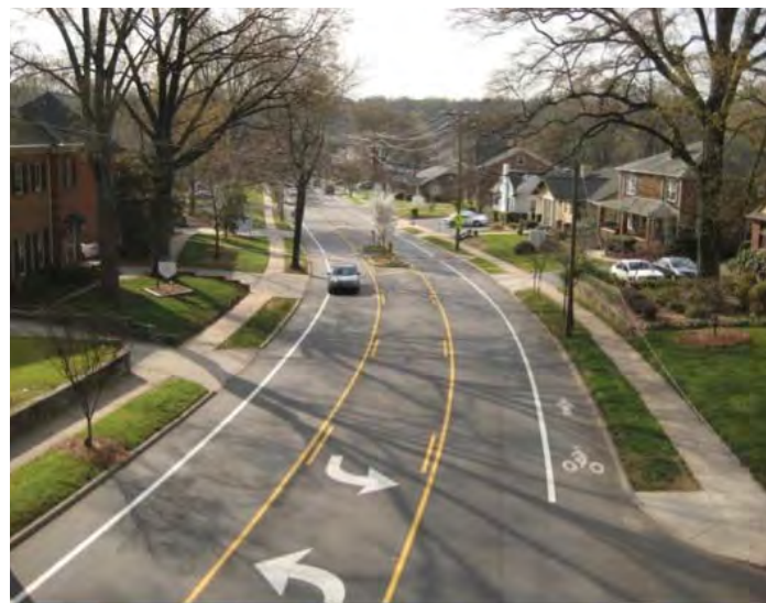
Example of a complete street design with center turn lane, bike lanes, and sidewalks in a residential neighborhood (Charlotte, NJ; Source: Charmeck.org)
