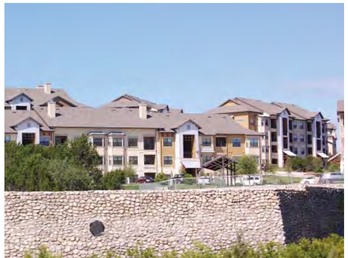
Multi-family housing under construction
