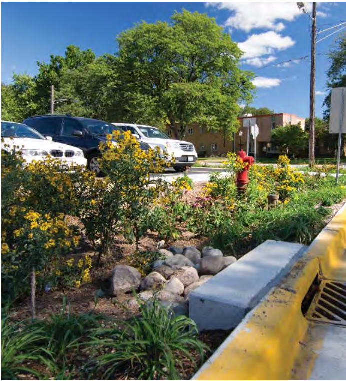
Stormwater runoff from a parking lot is delivered to a series of rain gardens to reduce runoff (CNT)
